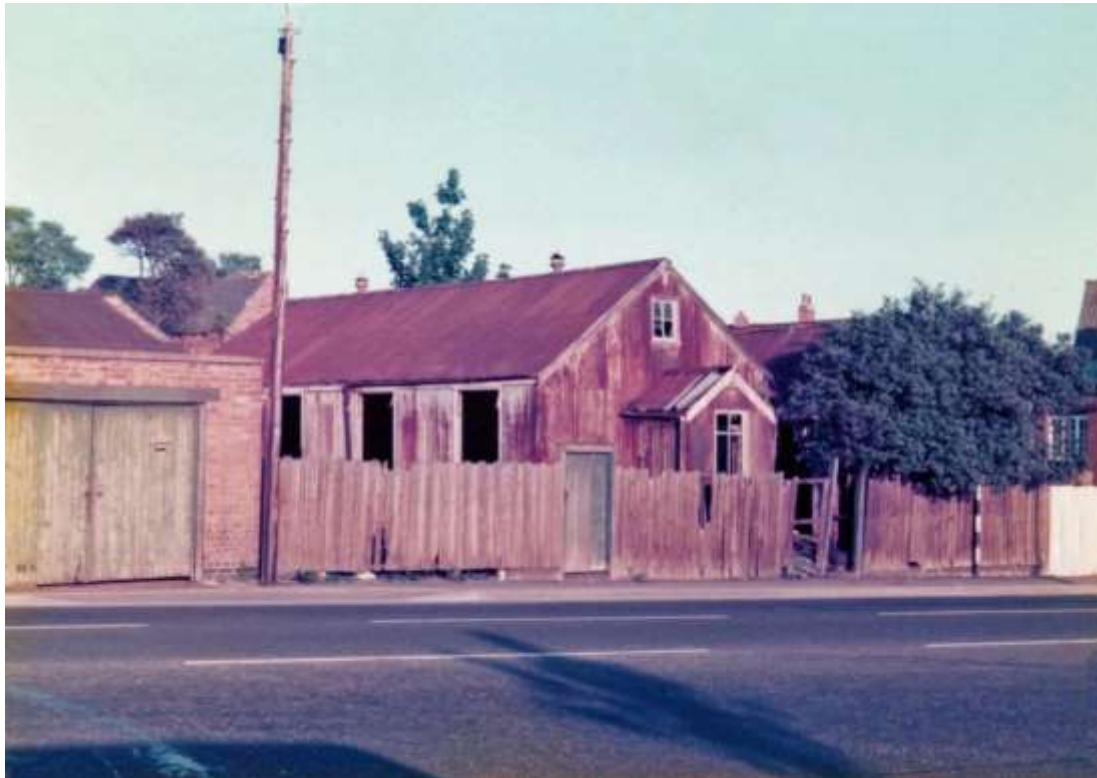
Wigston Adult School waiting to be demolished in the 1970s
